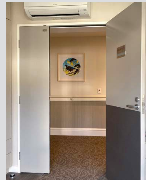
Wheelchair Access 1.5 Wide Doors
