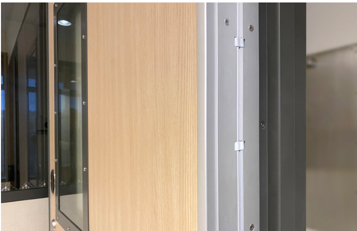
Hallmark doors with single swing anti-ligature hinges and anti-ligature tip at Burwood Hospital
