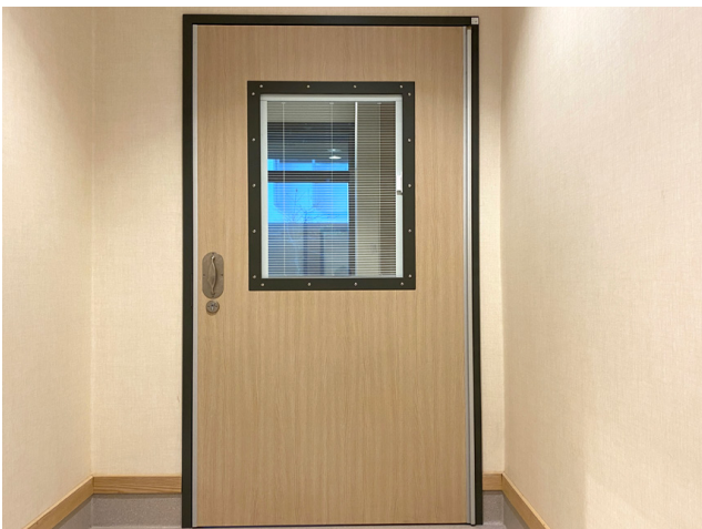
Hallmark seclusion room doors with security hardware at Burwood Hospital
