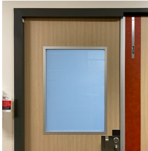
The same door with iGlass vision panel turned on
